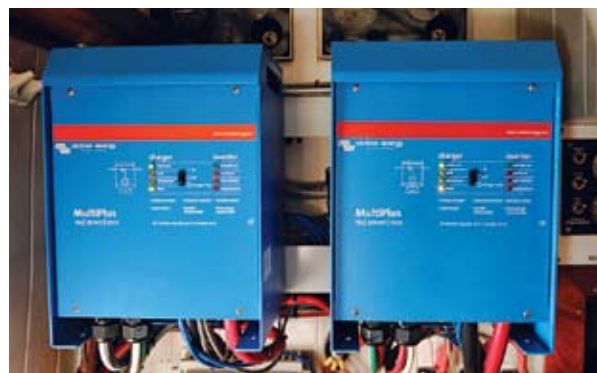
QUIET MORNINGS in places such as Canada's Rideau Canal (top) can now be enjoyed without the intrusive sound of a large generator. East Passage , under way near Baltimore (above center), couples alternators to a pair of Victron inverters to meet AC needs (above).
